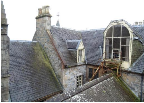
Attic studio fire escape (right)
