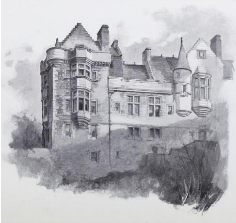
North elevation showing Leiper's additions which appears to include the oriel window of the original staircase (right)
