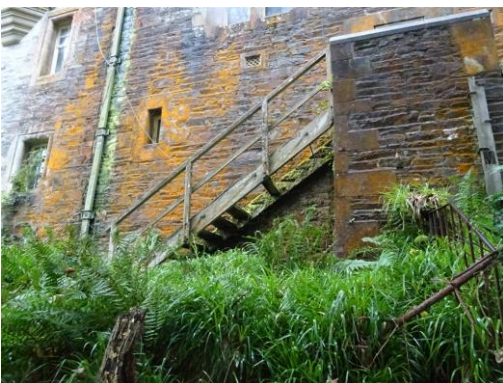
External existing timber staircase
