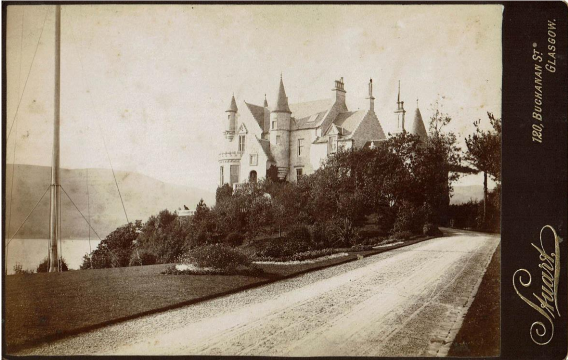
Undated photograph showing Knockderry Castle at Phase 3 of development. Note the absence of stained glass in the bow window, no dormer windows in the highest duo-pitched roof, the absence of the staircase below the largest corbelled turret and the absence of the later Leiperian Tower.
