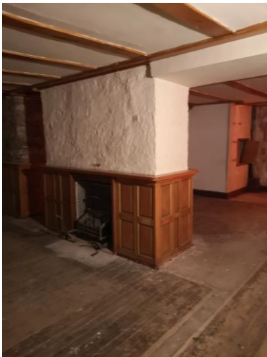
Wall at former bar
