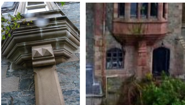
Oriel window with vertical support (Knockderry left and Craigrownie right)
