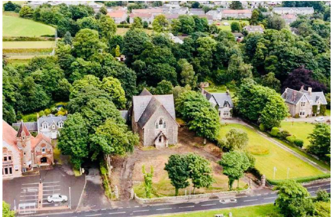
Drone Footage of the Church Hall
